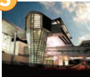
George Bush Intercontinental Airport now ranks third in the nation for domestic and international service to 170 destinations.
